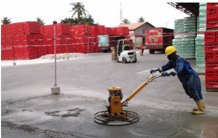
Monolithic floor hardener Arbico site, Cocacola Mushin
