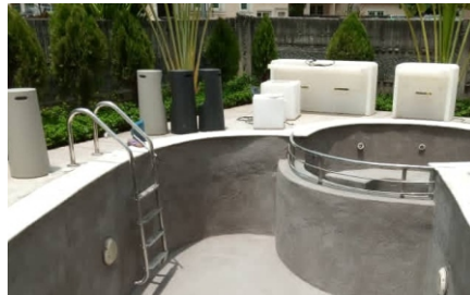
Waterproof fountain walls Shoreline, Ikoyi
