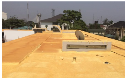
Flat roof Waterproofing Protea Hotel Lagos.
