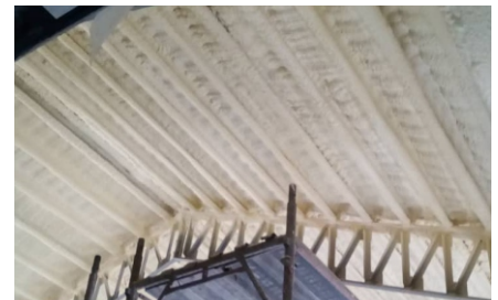
Roof Insulation Lekki Lagos.
