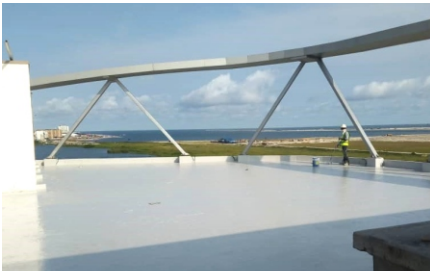
PU roof slab Waterproofing Charvet Construction
