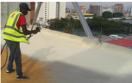
Roof waterproofing White Orchid Hotel, VI Lagos.
