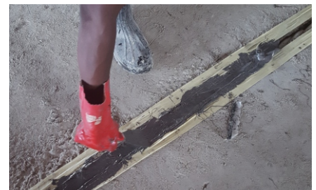
Expansion Joint Sealant Shapoorji, Lekki Phase 1
