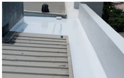
Polyurethane waterproofing Ponti Itaware site, VI Lagos.
