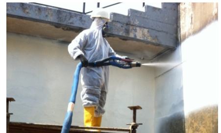
Polyurea coating Water corporation, Enugu
