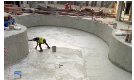
Swimming pool waterproofing Empire Court, Lekki
